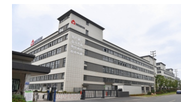
高新区工厂 High-tech zone site
